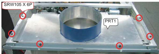
② Install the Bracket T and the Insulation Plate A.
