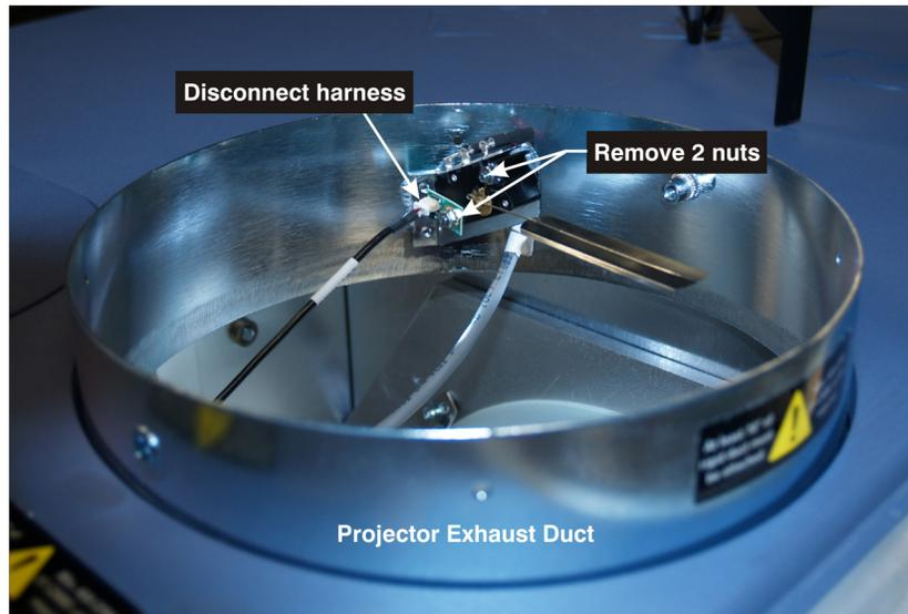
**FIGURE 1-61 EXHAUST DUCT VANE SWITCH**
