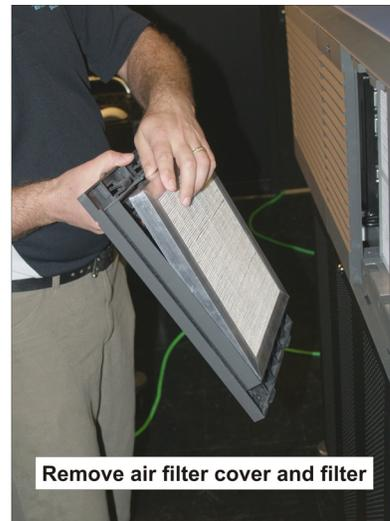
**FIGURE 1-11 REPLACING AN AIR FILTER**
